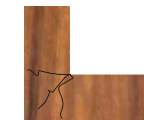
Cutting a laminate sheet at an angle of 90 degree leads to development of cracks. In corner after pasting. Therefore it is advisable to avoid cutting at an angle of 90 degrees.
